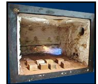
Small vessel stress relieved in temporary furnace.
